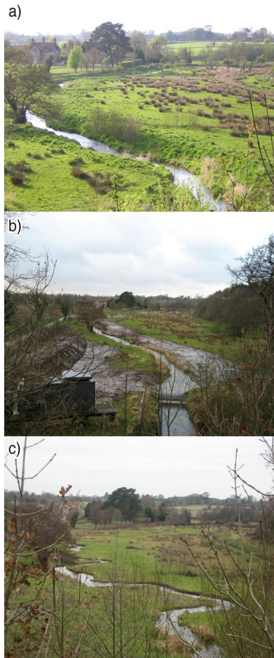
Fig. S1. Restoration reach of the River Glaven at Hunworth (north Norfolk, UK): (a) in January 2009, prior to the renaturation project; (b) after removal of embankments in March 2009; and (c) in December 2010, after recreation of meanders in August.
