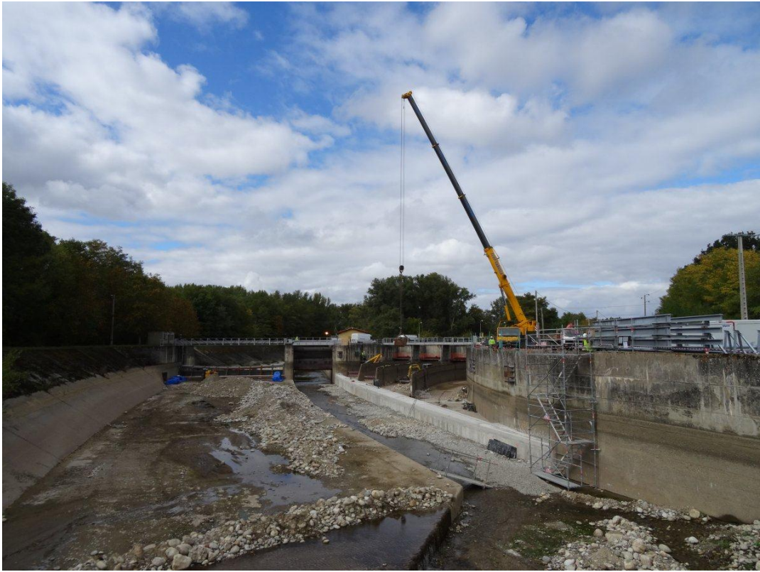
Figure 1: Picture of Pébernat fine-spaced rack during construction
